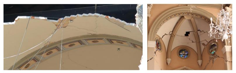
Fig. 12 – Examples of vault structures made of brick masonry laid flatwise in church I1.
