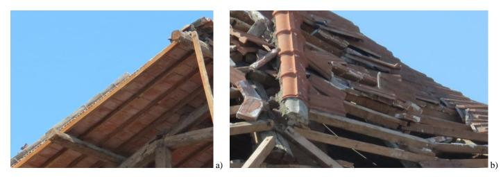
Fig. 11 – Example of roof sheeting made of hollow masonry elements in church I9 (a), and made with solid masonry elements in church I3 (b).
