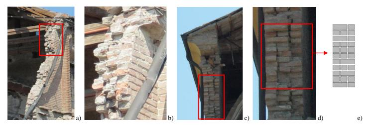
Fig. 8 – Irregular triple header brick masonry bond in church I9, general view (a) and detail (b), and in church I10, general view (c) and detail (d), and sketch of the highlighted part of the cross section bond (e).
