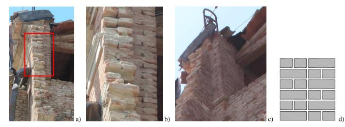
Fig. 5 – Double wall made of double header brick masonry bond in church I1: general view (a), detail (b), view from the back side which supports a timber truss (c) and sketch of the cross section of the duplicated wall in the region of the truss support (d).
