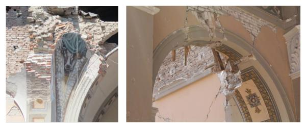
Fig. 15 – Examples of arches made of vertically stacked brick masonry in church I1.
