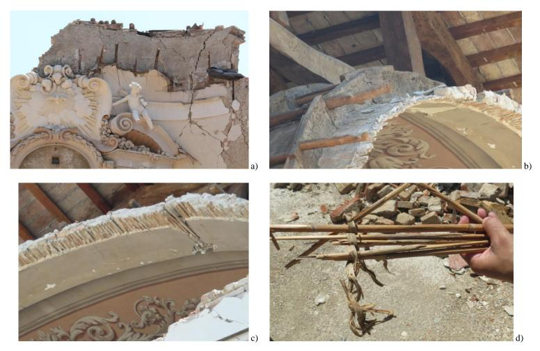
Fig. 13 – Examples of reed mat false vaults in churches I2 (a) and I10 (b) and (c), and detail of a reed mat (d).
