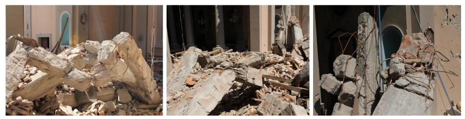
Fig. 17 – Collapsed reinforced concrete beam in church I1.
