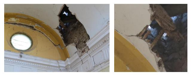
Fig. 14 – Example of a vault made of timber elements imbedded in mortar/plaster in church I11.
