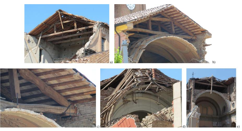
Fig. 10 – Examples of roof structures made of timber trusses in churches I9 (a), I10 (b) and (c), I3 (d), and I1 (e).
