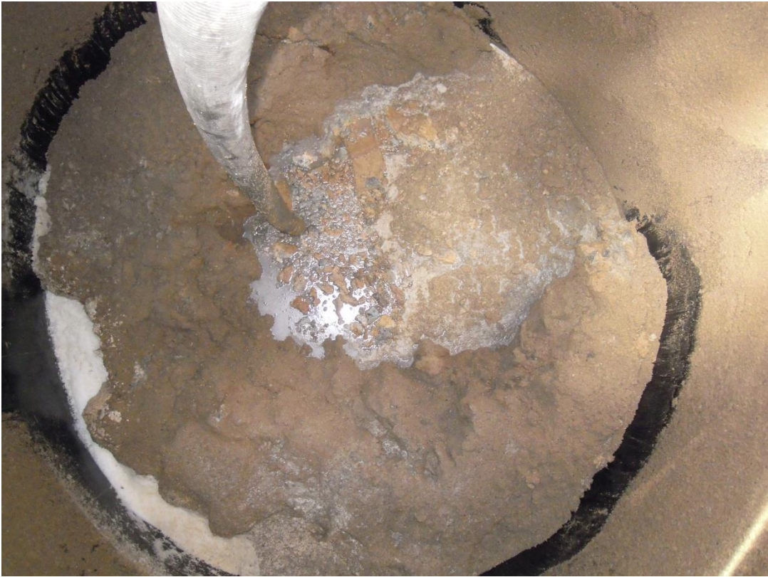
Figure 21: Equalization Tank (T102) and the solified fat layer.
