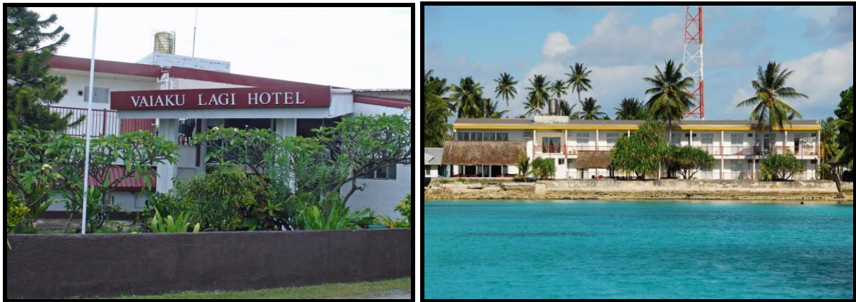
Figure 22 The Vaiaku Lagi Hotel: Front view and lagoon view (Source: Niko Iona )
