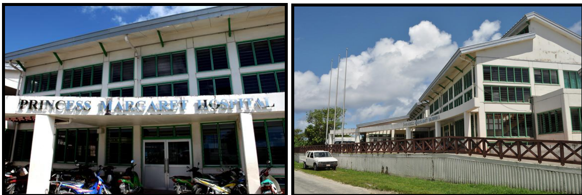
Figure 31 Princess Margaret Hospital, Tuvalu's only hospital (Source: Niko Iona )
