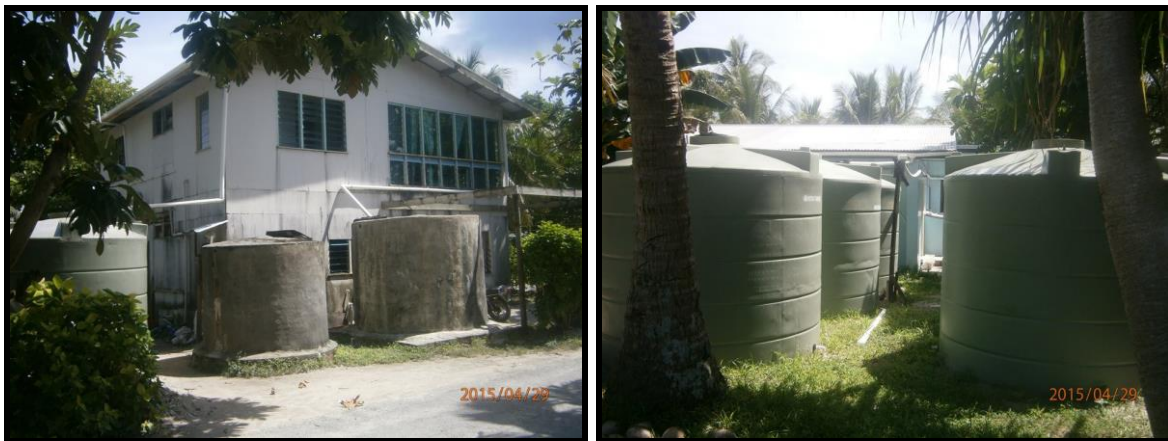
Figure 29 Houses surrounded by water storage tanks at Funafuti, Tuvalu (Source: Niko Iona )
