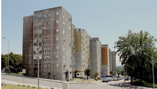
Before the architectural engineering in rehabilitation
