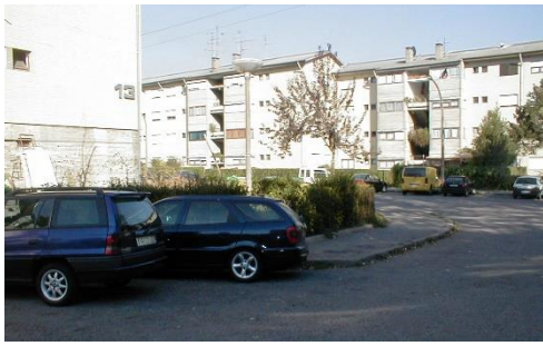
Before the architectural engineering in rehabilitation
