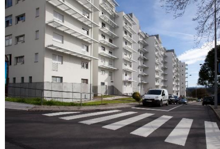
After the architectural engineering in rehabilitation
