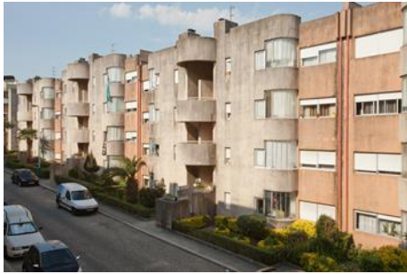
Before the architectural engineering in rehabilitation
