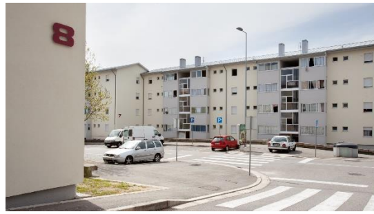
After the architectural engineering in rehabilitation
