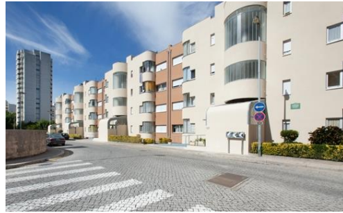
After the architectural engineering in rehabilitation
