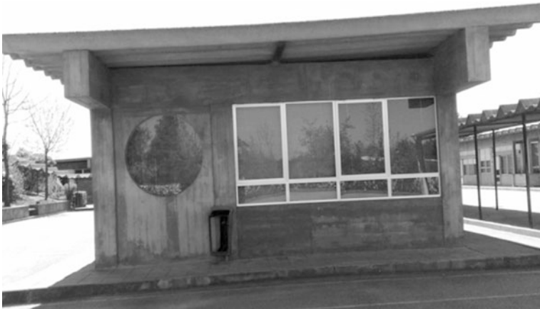
Fig. 3 School building's north façade
