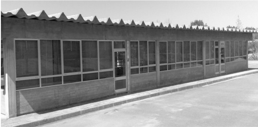
Fig. 2 School building's East façade
