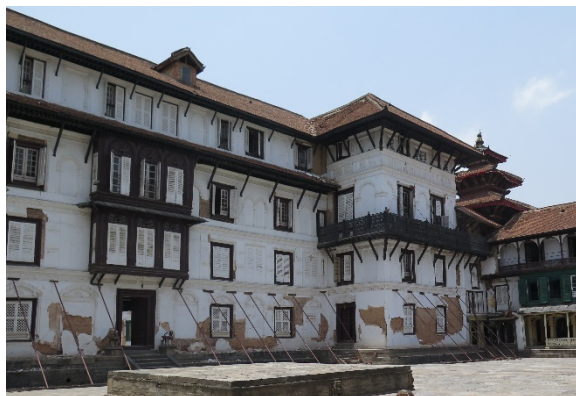
Figure 13 – View of the damages in façade 2 of Hanuman Dhoka and of the shoring structures
