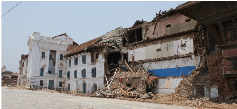
Figure 19 – View of the damages in façade 4 of Hanuman Dhoka and view of the interior wall of the building in the section of the façade that collapsed during the earthquake
