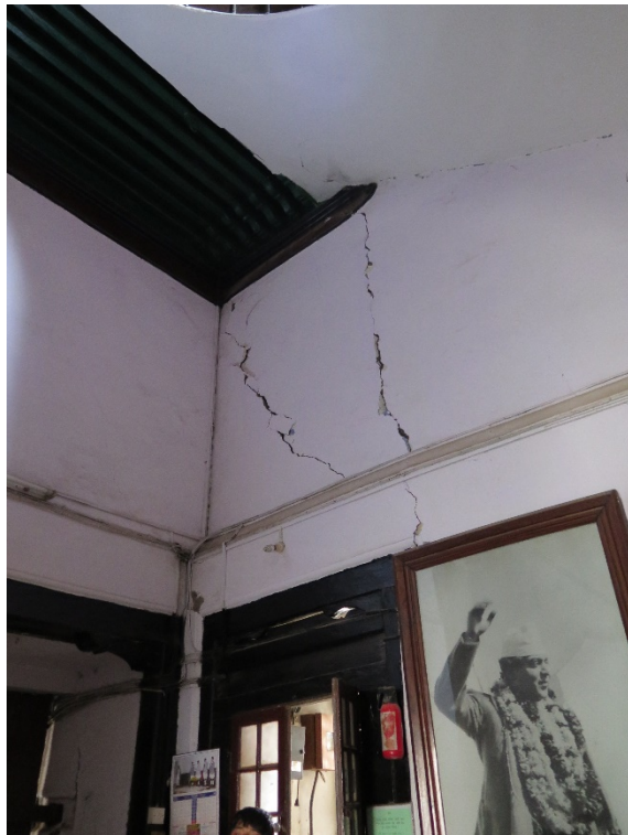
Figure 34 – Cracks visible in the top part of one of the ground floor wall
