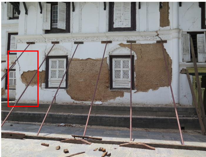
Figure 5 – Cracks and delamination in the mortar layer
