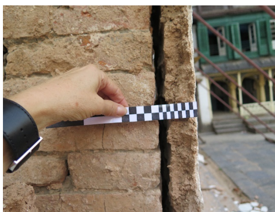
Figure 2 – Mortar layer of the walls with 4 cm thickness currently detached 1 cm from its support
