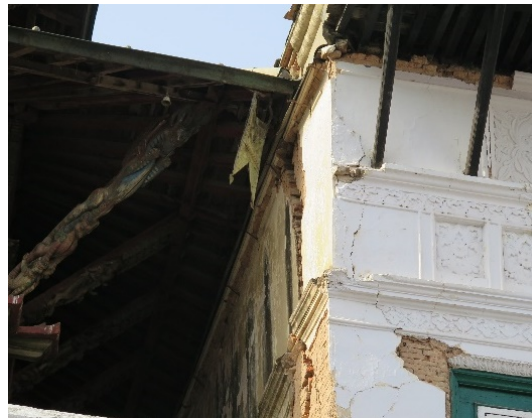
Figure 28 – View of the damages in façade 9 of Hanuman Dhoka
