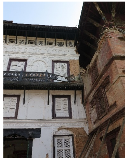
Figure 12 – View of the damages in façade 1 of Hanuman Dhoka and of the shoring of the Deutaleju temple
