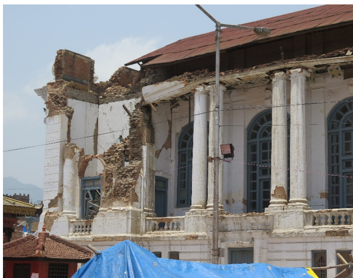
Figure 22 – View of the damages in façade 5 of Hanuman Dhoka
