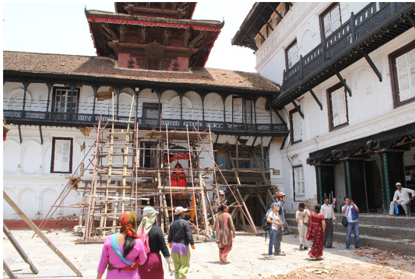
Figure 10 – View of the entrance of Hanuman Dhoka which is shored due to its level of damage
