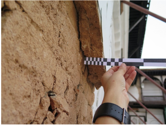
Figure 3 – Mortar layer of the walls with 5 cm thickness
