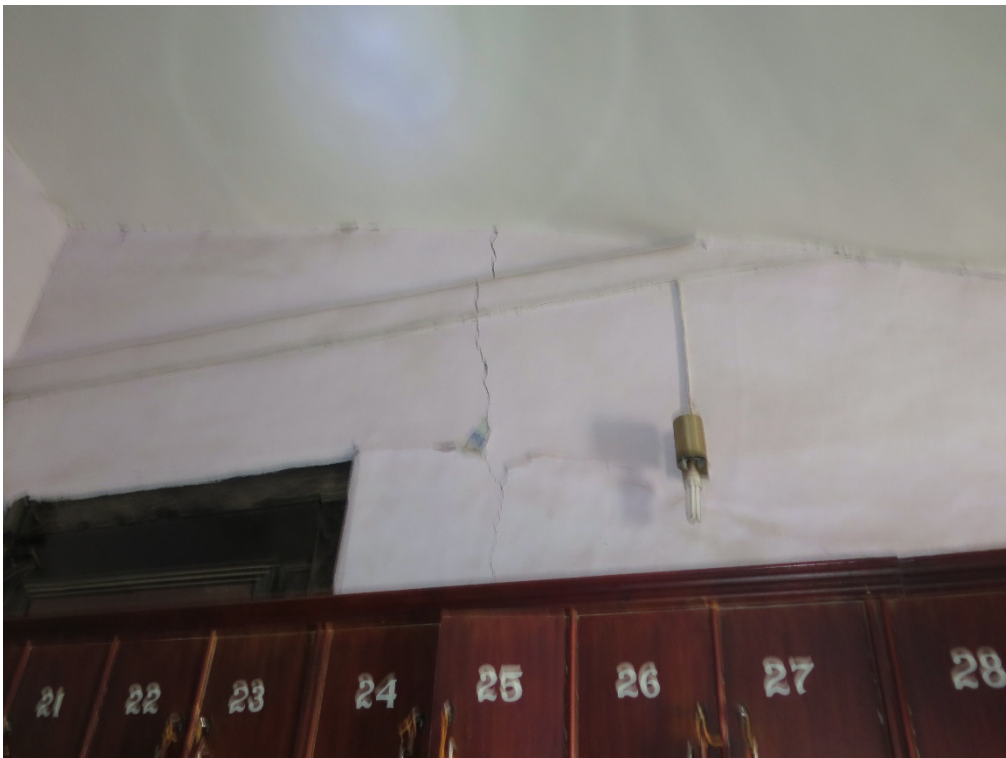
Figure 37 – Cracks visible in the top part of one of the ground floor wall
