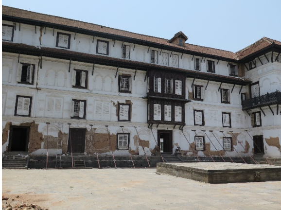
Figure 15 – View of the damages in façade 2 of Hanuman Dhoka and of the shoring structures
