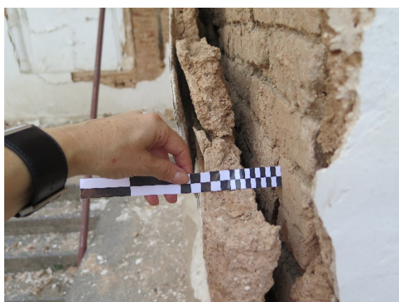
Figure 1 – Mortar layer of the walls with 4.5 cm thickness currently detached 3 cm from its support
