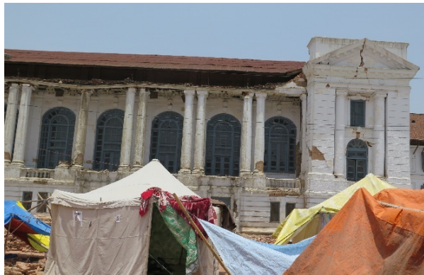
Figure 20 – View of the damages in façade 5 of Hanuman Dhoka
