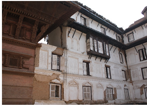
Figure 18 – View of the out-of-plane deformation of façade 3 of Hanuman Dhoka and view of the out-of-plan damage of the lateral exterior wall of the building that is currently partially supported by the Nautalle temple
