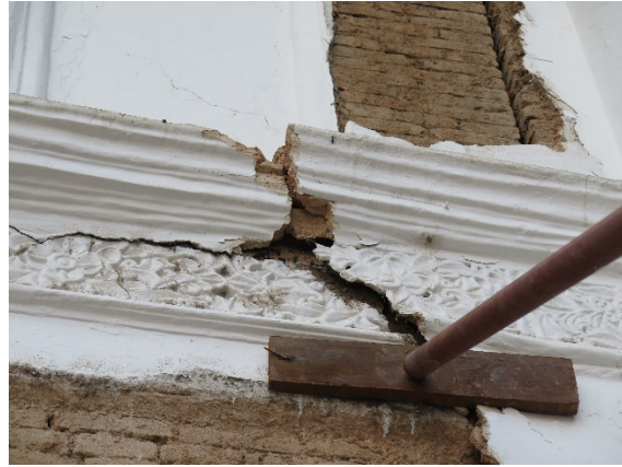
Figure 4 – Cracks in the decorative mortar layer
