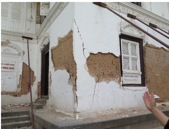
Figure 7 – Cracks and delamination in the mortar layer
