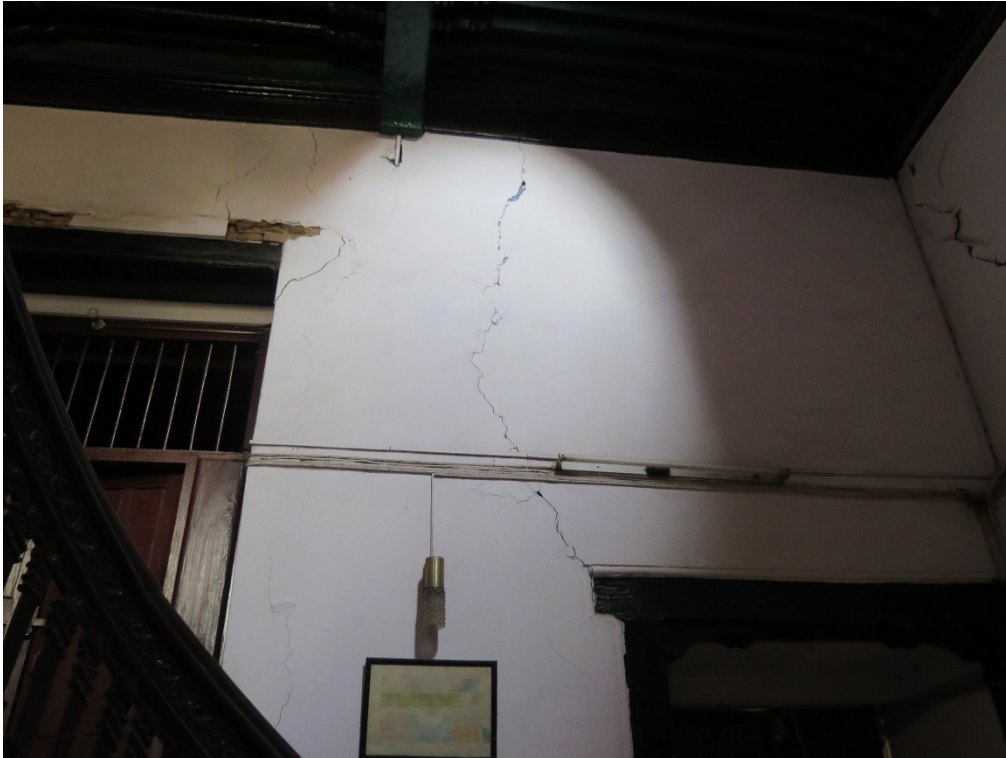
Figure 36 – Cracks visible in the top part of one of the ground floor wall
