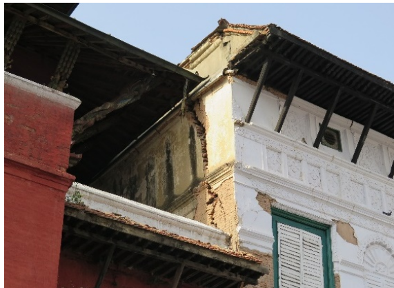
Figure 27 – View of the damages in façade 9 of Hanuman Dhoka
