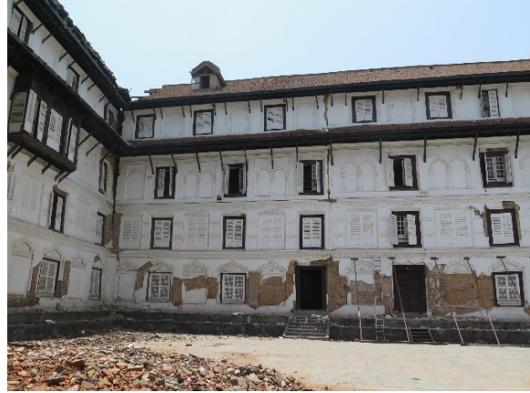
Figure 16 – View of the damages in façade 2 of Hanuman Dhoka and of the shoring structures
