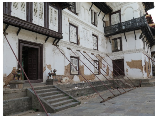
Figure 14 – View of the damages in façade 2 of Hanuman Dhoka and of the shoring structures
