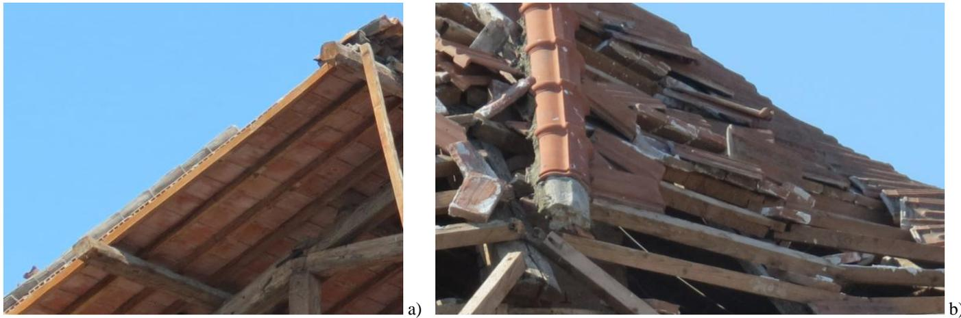
Fig. 11 – Example of roof sheeting made of hollow masonry elements in church I9 (a), and made with solid masonry elements in church I3 (b).
