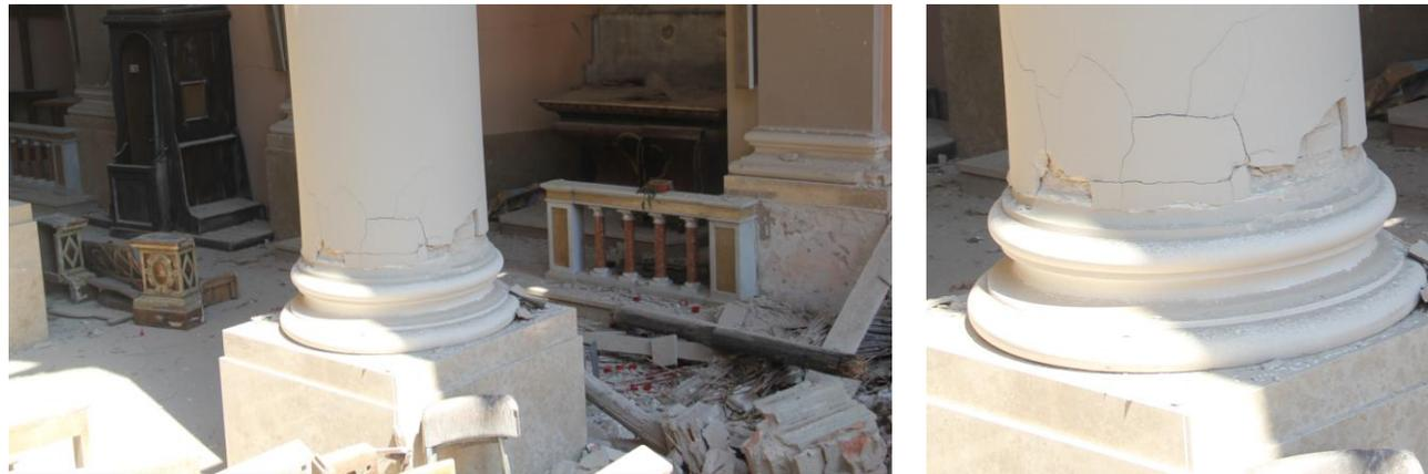
Fig. 16 – Example of an interior column made of brick masonry in church I1.
