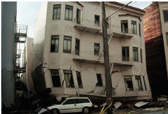
c) A collapsed soft storey apartment building in the Marina District, San Francisco 1989 (Loma Prieta Earthquake) [4]
