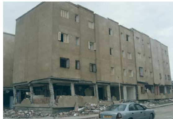
d) Damage to an apartment building with a soft first storey in Bordj-Kiffan city, Algeria 2003 [5]
