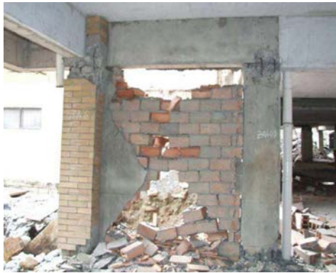
a) Infill shear and major frame damages, Chania 2008 [3]
