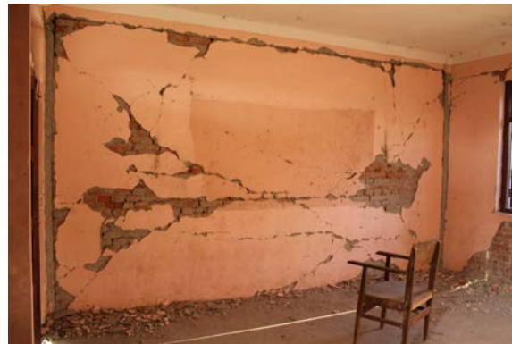
b) Infill shear and minor frame damages, Nepal 2015
