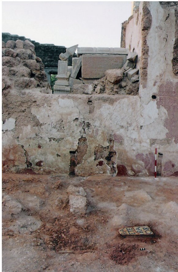
Fig. 6. Church of Our Lady of Grace, Old Goa, built 1597–1620, view of the Chapter room and the window with the urn of Fr. João da Cruz (Siddh Lasa Mendiratta 2006).
