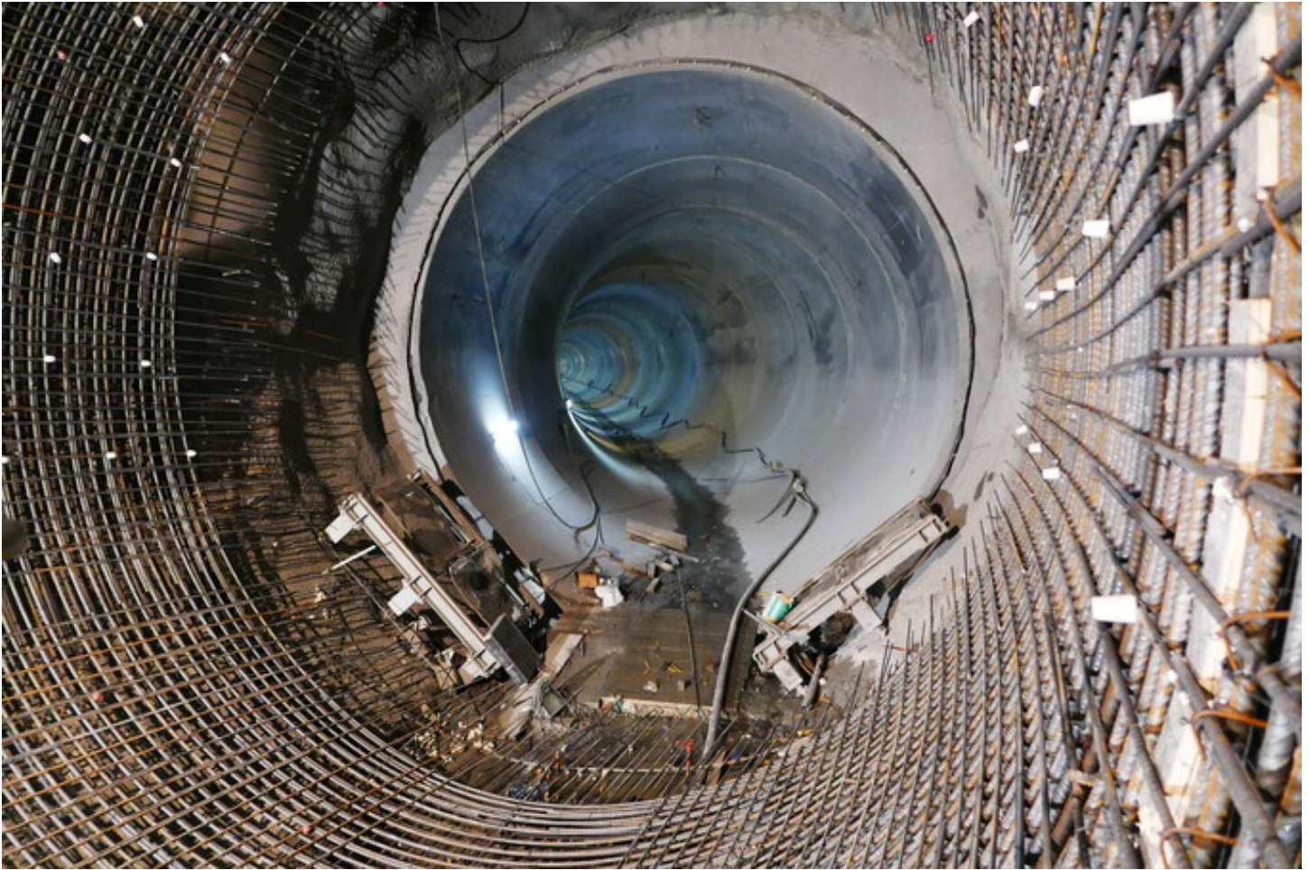
Vertigo. Pressure pipeline for passage of water between reservoirs, 2022. © Alvaro Domingues.
