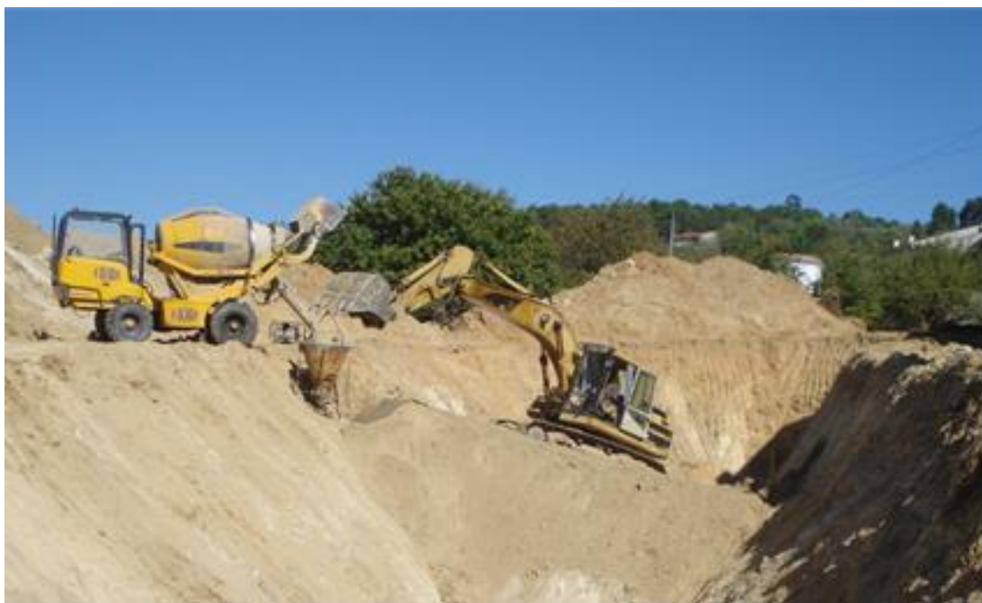
Figure 6. Certified equipment used on site (Henrique, 2017).
