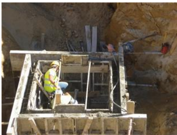
Figure 8. Prevention in the execution of the formwork and concreting of a mine visit box (Henrique, 2017).
