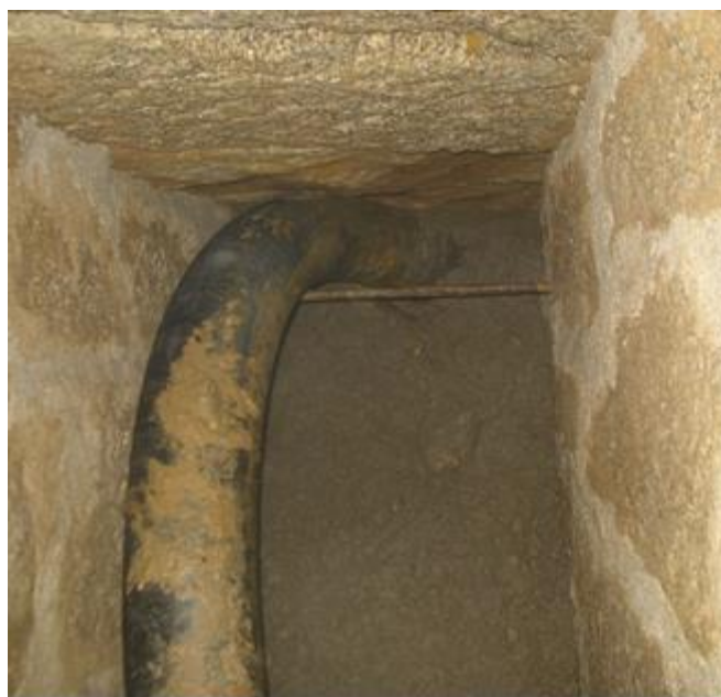
Figure 5. Concrete pump for mine buffering (Henrique, 2017).
