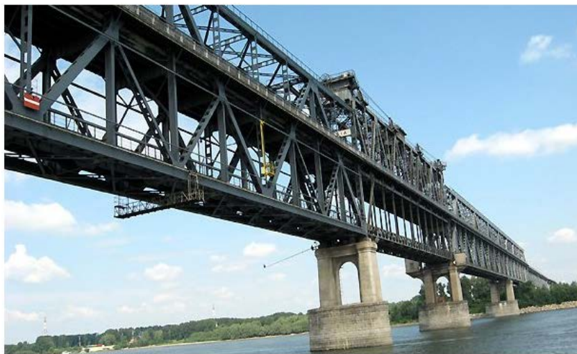
Fig. 4. The Danube Bridge, the town of Ruse.
