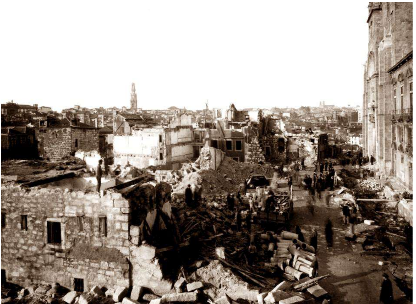
Aspect of the demolitions, for the extension of the Terreiro of D. Afonso Henriques, current Terreiro da Sé.
