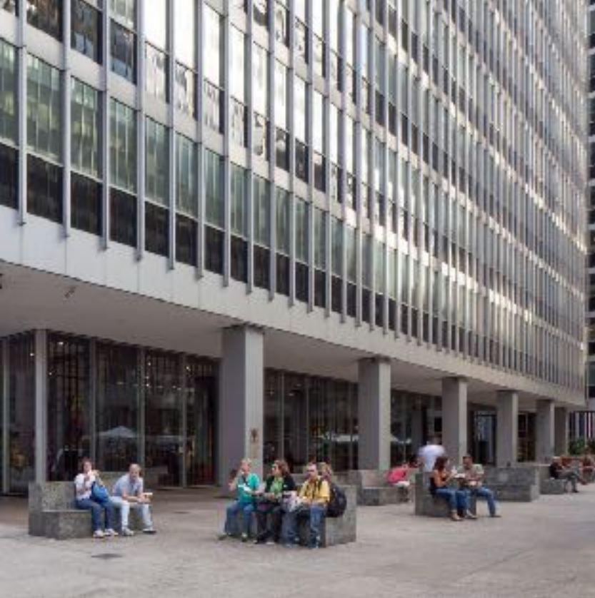
Fig. 1. Vista do Google Street View da obra 'Urban Plaza North', localizada na Avenida 52, Nova York, 2022 © Google Street View.
