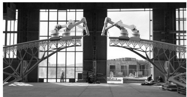
Fig. 1. 3D-printed steel bridge [1]
