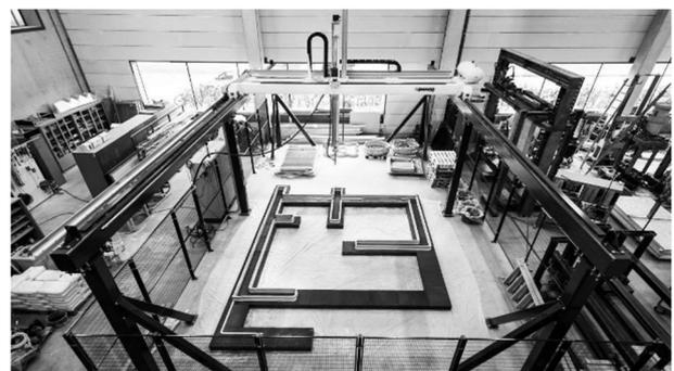
Fig. 2. 3D-printed concrete house [2]
