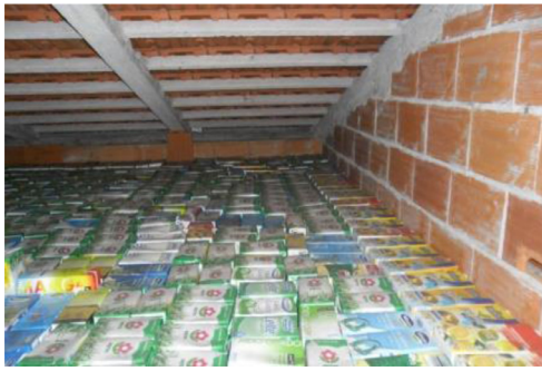
Fig. 5. Application of empty liquid food cartons on the floor of the roof attic.
