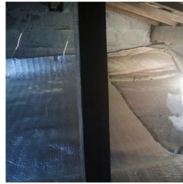
Fig. 13. Inside the attic of the eastern roof during the application of the radiant barrier.
