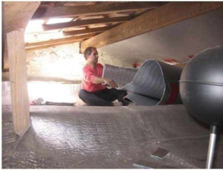
Fig. 15. Application of radiant barriers under the eastern roof slopes.
