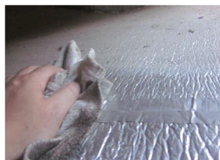
Fig. 28. Dust had accumulated on the radiant barrier applied in the summer of the 1st year.
