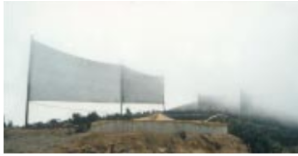
Figure 2.5. Typical fog water collector with fog harvester arranged in the perpendicular direction of the wind [59].
