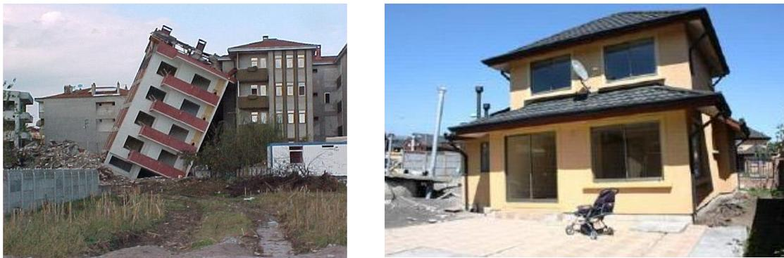
Figure 1 – Damage in structures due to soil liquefaction: a) bearing capacity failure; b) differential settlement.
