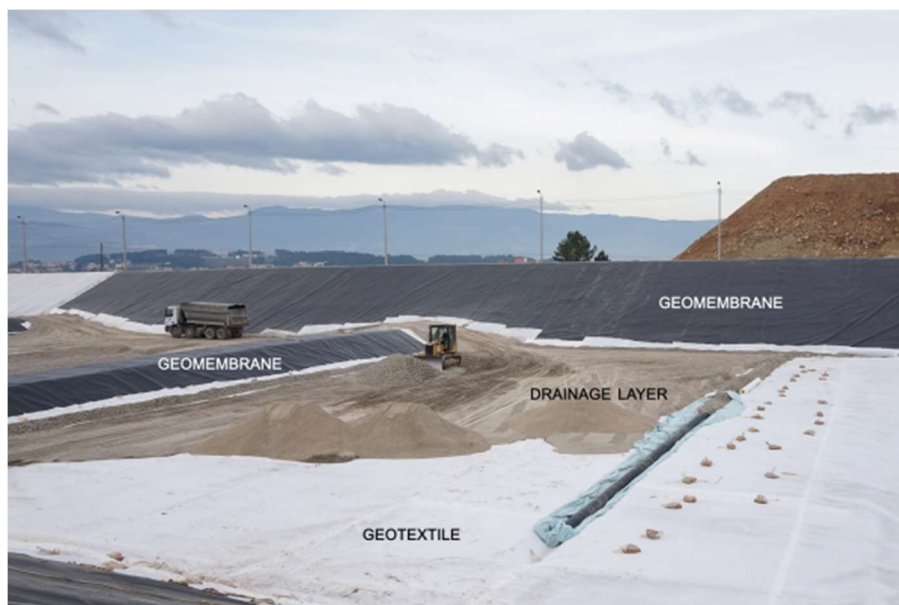
Base liner system of a waste landfill.
