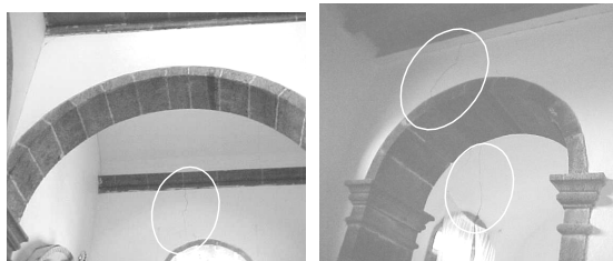
a) Crack between the windows and the coping
