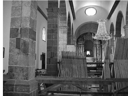
Figure 3 Arches supporting the lateral and central naves
