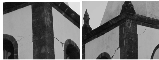
a) Cracks around the towers
