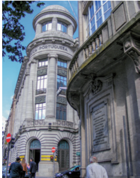
[319] - (Previous page) - photography with a view to a set of rounded corner buildings, being in the 1 st plan the building of 'Caixa Geral de Depósitos'. (VALE, 2013)
