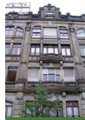
Group of buildings Liberdade Square 62-68 c.1930
