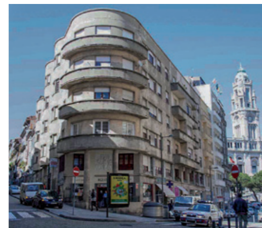
[428] - Corner of 'Soares Marinho' building, showing the sharp difference of levels between the two streets. (LIMA, 2013)
