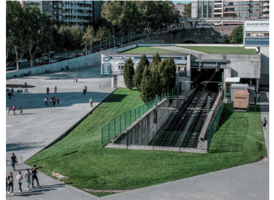
[192] - The Porto Metro Station – Trindade - Eduardo Souto de Moura project, 2012 (PINHEIRO, 2012)
