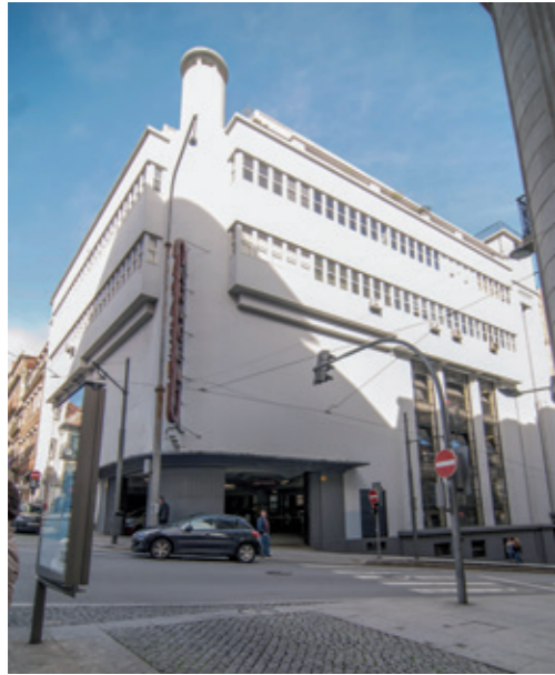
[347] - Current View of the round corner of the Garage of 'O Comércio do Porto'. (BENTO, 2013)
