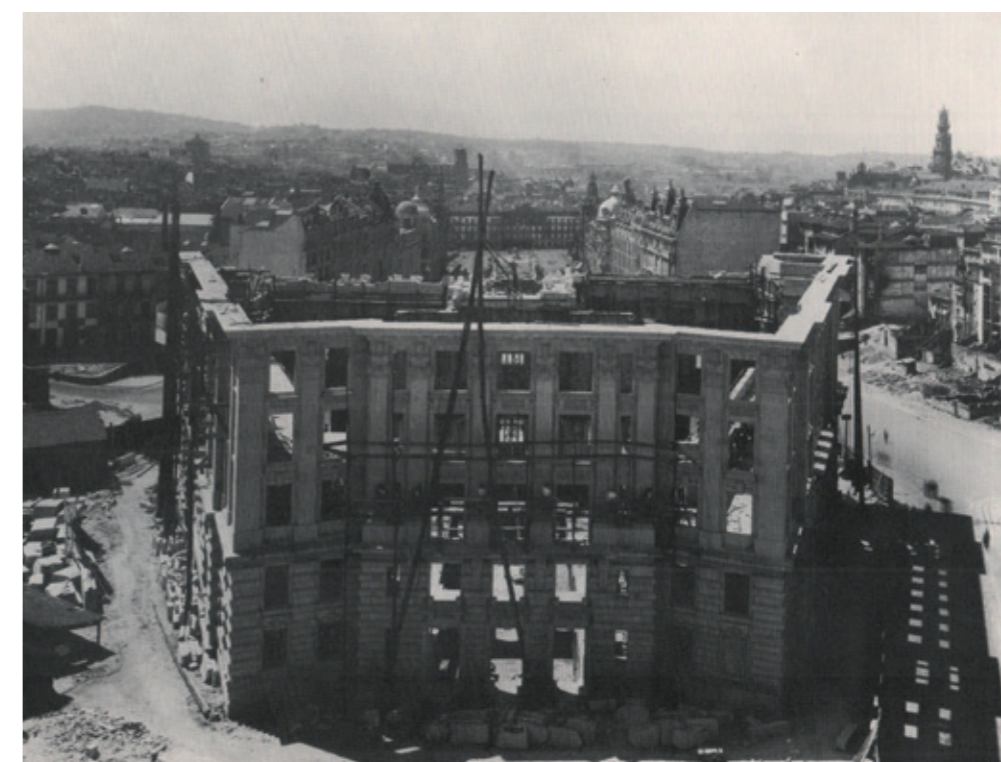
[210] - Start of demolitions. West Side of Laranjal Street, already completely demolished (1916-1917), of Aurélio Pais dos Reis. (DIAS & MARQUES, 2002)
