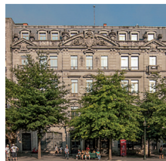
[236] - BNU Building. Noted the mansard changes in relation to photography of the 1930s. (BENTO, 2013)
