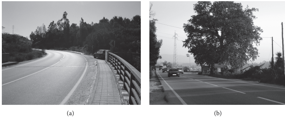
FIGURE 1: Examples of the considered roads: N 101 (a) and N 206 (b).
