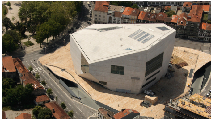
Figure 12 – Rem Koolhaas Casa da Música, aerial view. Clara Pimenta do Vale, 2008. A real architectural diamond that crowns the program of the European Capital of Culture 2001.
