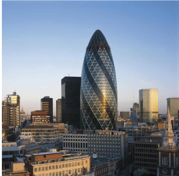
Figure 24: Photo of Gerkin Tower in London (Mutuli, 2022)
