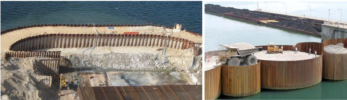
Figure 2.10 - Example of double wall tie cofferdam (left) and cellular cofferdams (right) (C.J. Mahan)
