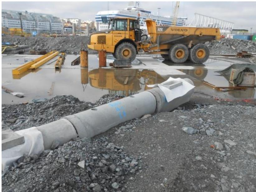
Figure 2.17 - Drainage system installed before applying top layer of filling material
