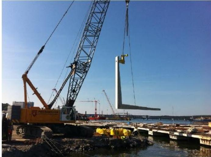
Figure 2.3 - Lifting of a gravity L-wall for positioning on-site
