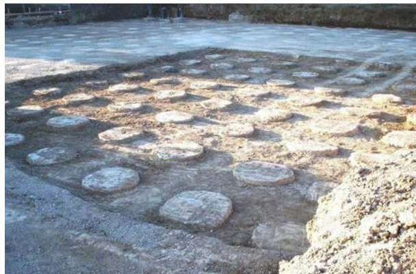
Fig. 26 – Colunas de Deep Soil Mixing (RAITO, Inc., 2023)
