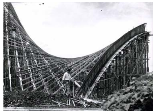
Scaffolding and formwork close-up
