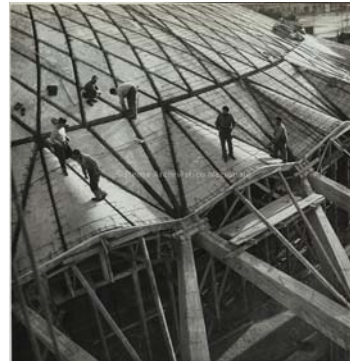
Rhomboid elements during construction
