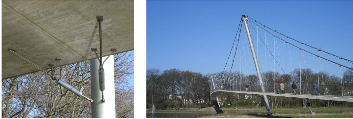
Figure 6-1: Example of viscous dampers
