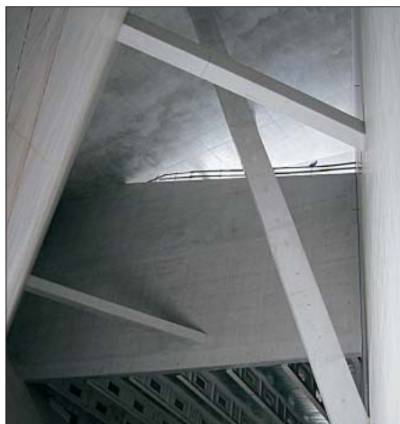
Fig. 2: Inclined column in South foyer
