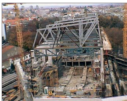
Fig. 7: Steel trusses in restaurant area
