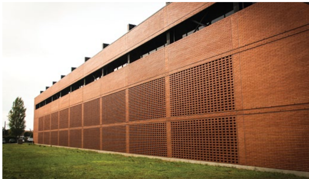
Departamento de Engenharia Civil, Projeto de Ana Reboredo e Joaquim Oliveira. Foto: CPV. / Department of Civil Engineering, Porto University, authored by Ana Reboredo and Joaquim Oliveira. Photo credits: CPV.
