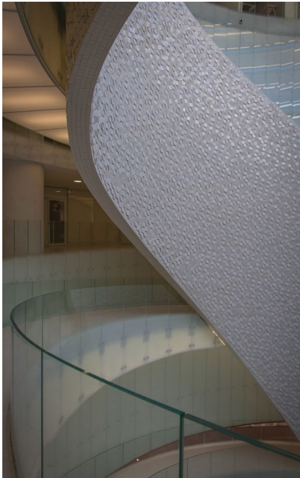
Vista da rampa circular interior e parede curva de suporte, igualmente revestida com o módulo cerâmico. Foto. CPV. / View of the circular ramp, and of the curved bearing wall, also covered with the ceramic hexagonal tile. Photo credits to CPV
