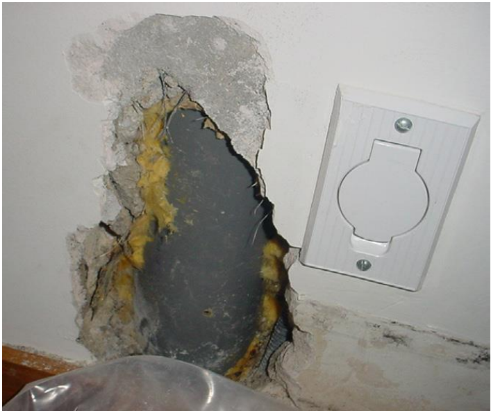
Figure 5.20. Detail of Courete in dwellings insulated with mineral wool.
