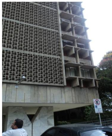
Fig. 4 – Cobogó on front of block services 206, Super Block North – Brasília – Distrito Federal (ARAÚJO, SIMÕES & SPOSTO, 2012) [14].
