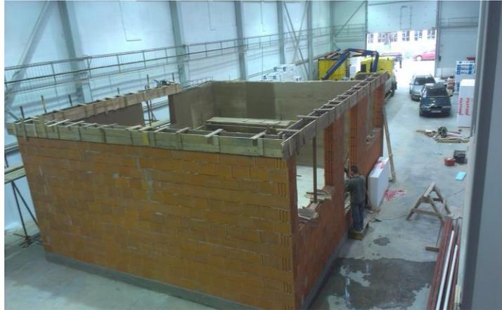
Fig.6 – Erection of the VUKONZE Climate chamber envelope.
