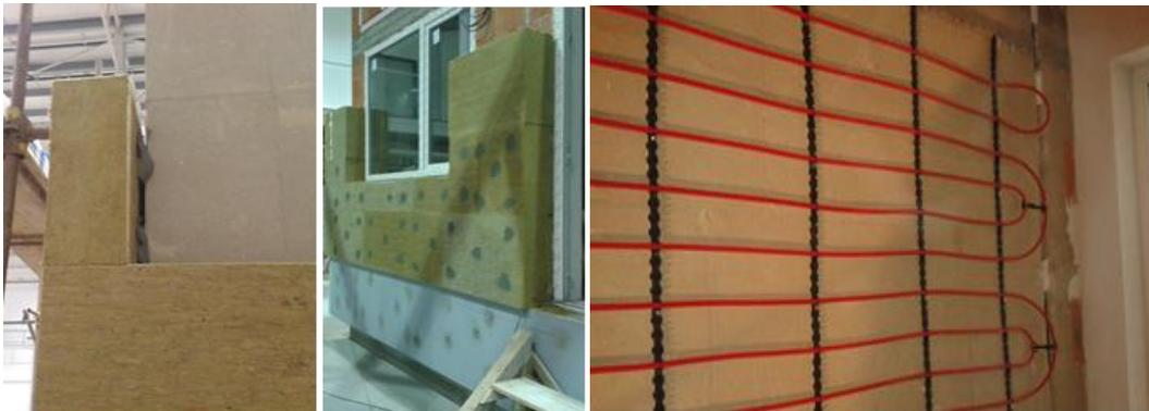
Fig.8 – Details of the VUKONZE Climate chamber additional insulation and wall heating system.
