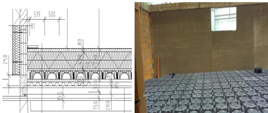
Fig.7 – Proposal and real construction of the VUKONZE Climate chamber floor.
