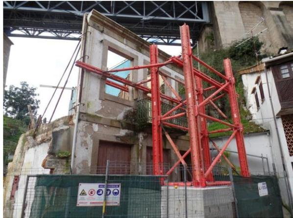
Fig.1 – Building facade with the respective containment.
