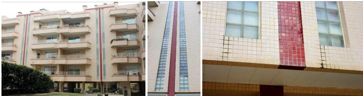
Fig. 4 – Configuration of the glass brick structures under study.
