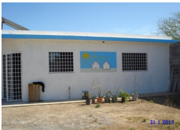
Fig. 4 Outside view of the prototype house.
