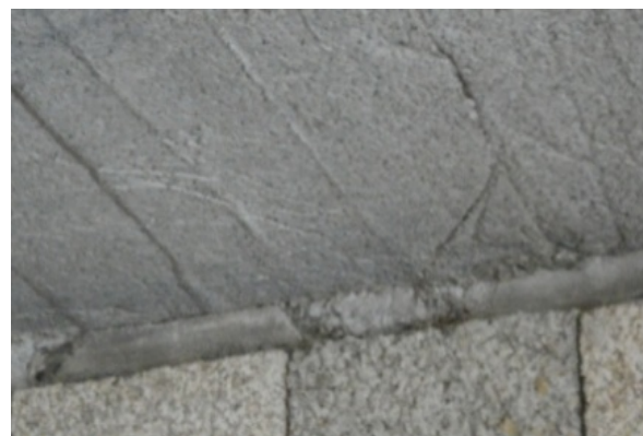
Fig. 5 Interior corner showing wall and roof interface.
