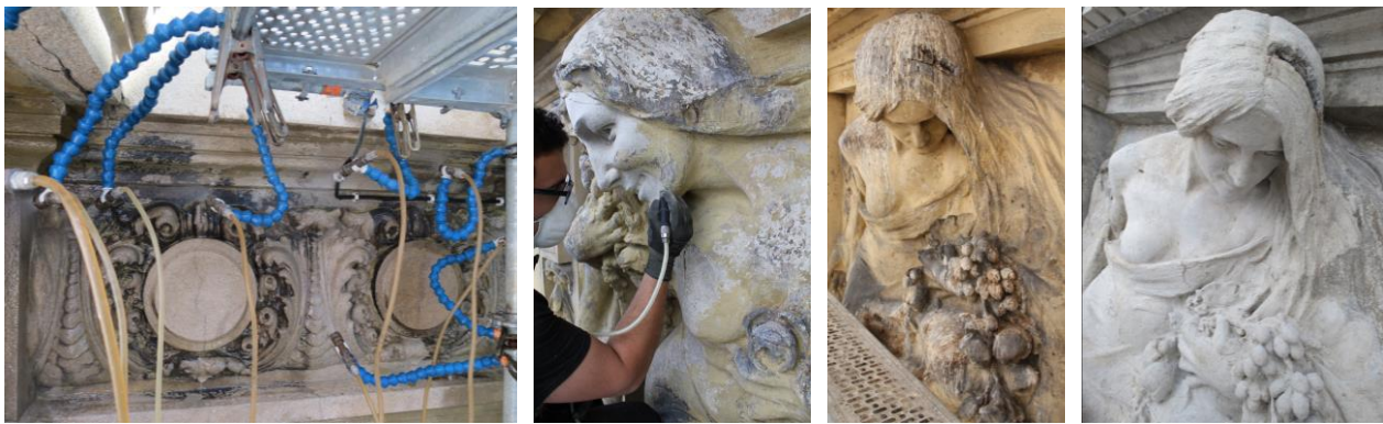
Figure 4 – Cleaning operation to remove limewash (left), cleaning operation by micro-abrasion (centre left), example of a decorative element before (centre right) and after (right) the cleaning operation.
