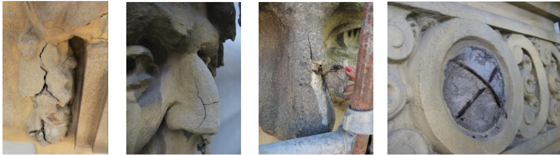
Figure 1 – Examples of reinforced concrete decorative elements and sculptures exhibiting some level of material degradation.
