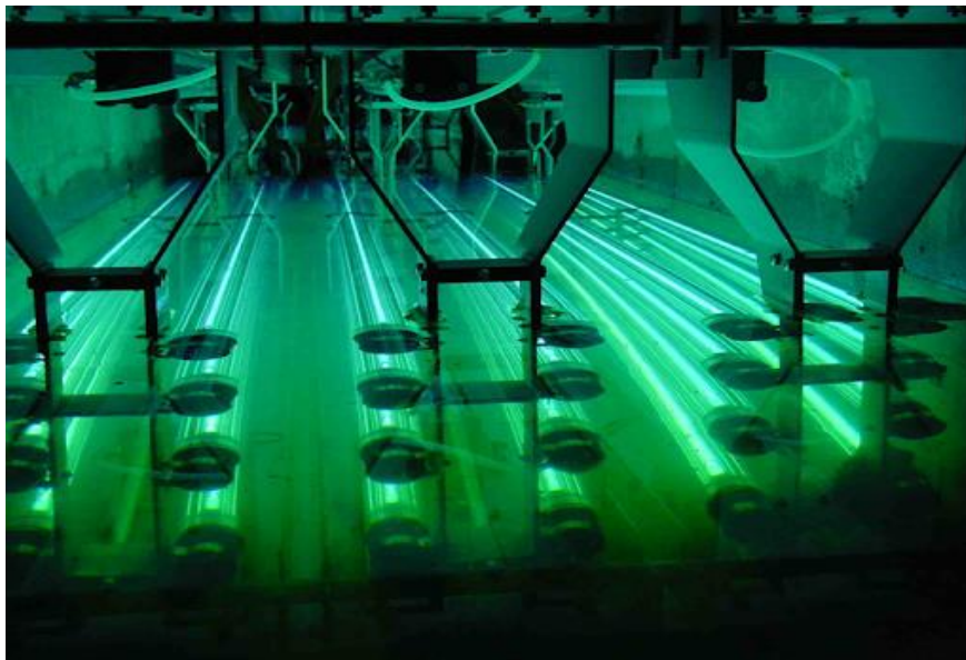
Figure 18: Example of UV lamps used for disinfection (water and Wastewater, 2020).
