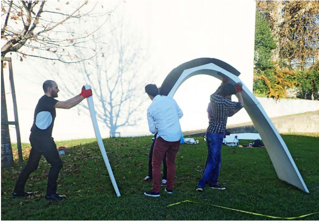
14 Assembly of the GRC panels.
