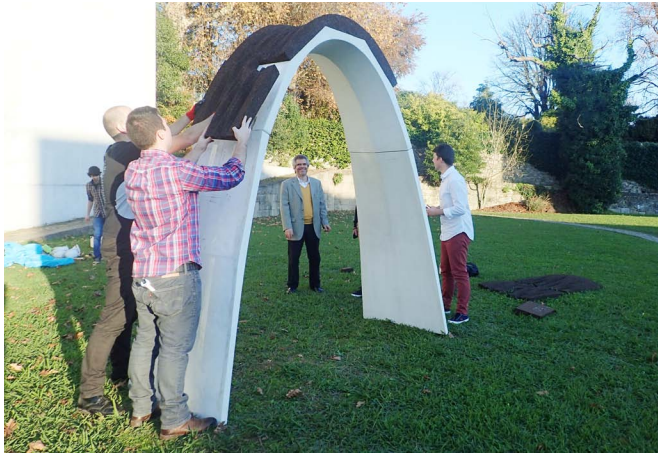
15 Fixation of cork panels.
