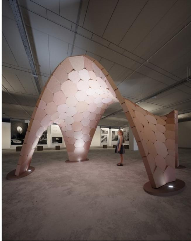
Prototype of earth voussoirs vault, as proposed to be installed in CCB/Garagem Sul.
