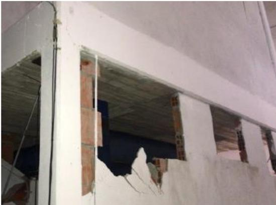
Fig. 3.22 – Partial collapse of the infill opening (ISAAC technical report, 2020)
