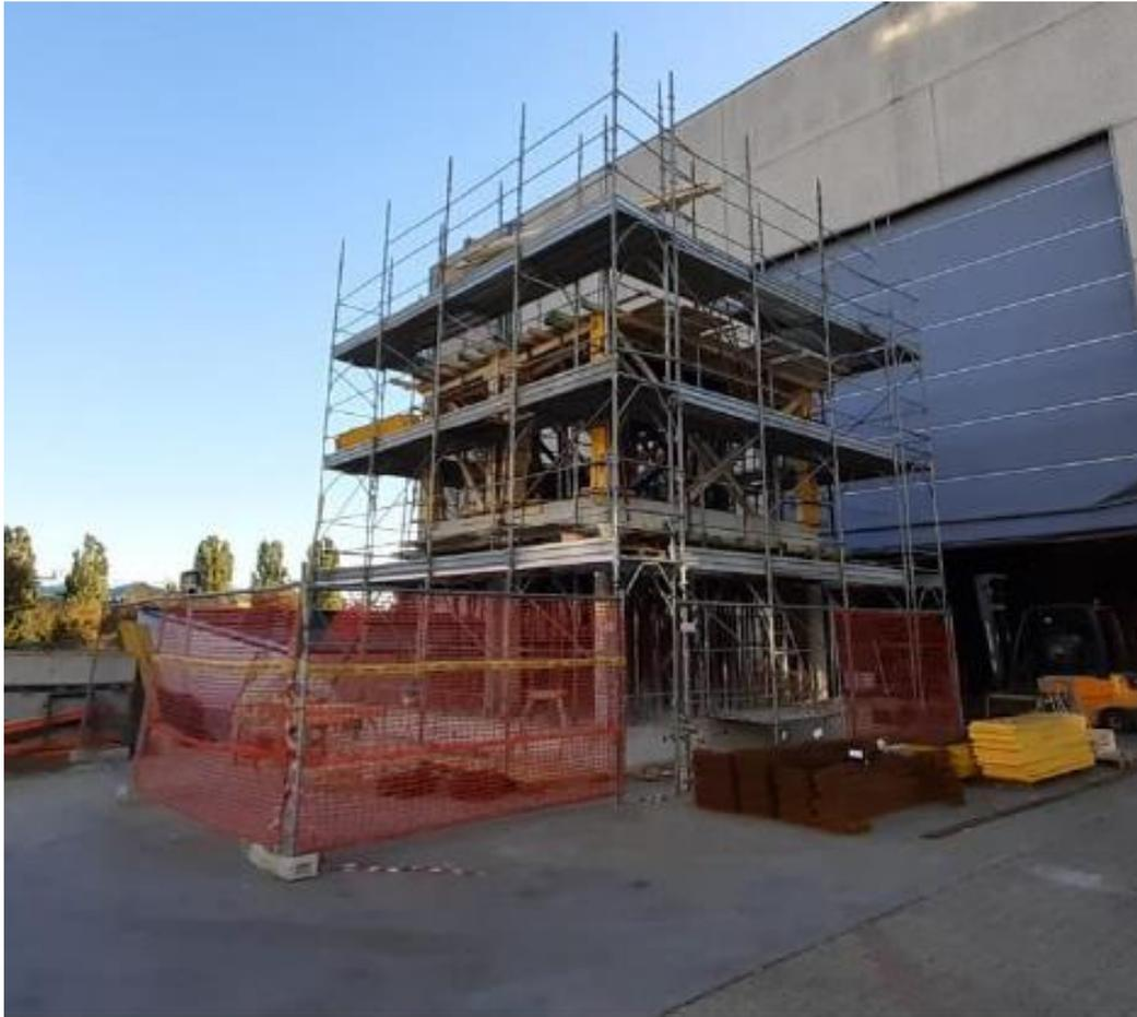
Fig. A.1 – Casting of the 2nd storey (general view) at the external area of the EUCENTRE laboratory (ISAAC technical report, 2020)
