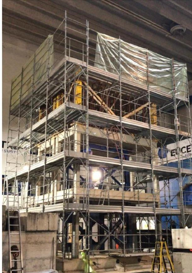
Fig. A.4 – Casting of the 3rd storey of the specimen structure (ISAAC technical report, 2020)
