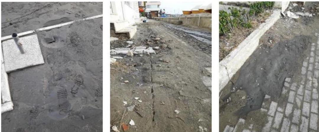
Fig. 2.6 - Liquefaction phenomena in the coastal part of southern Durrës (Andonov et.al., 2022)
