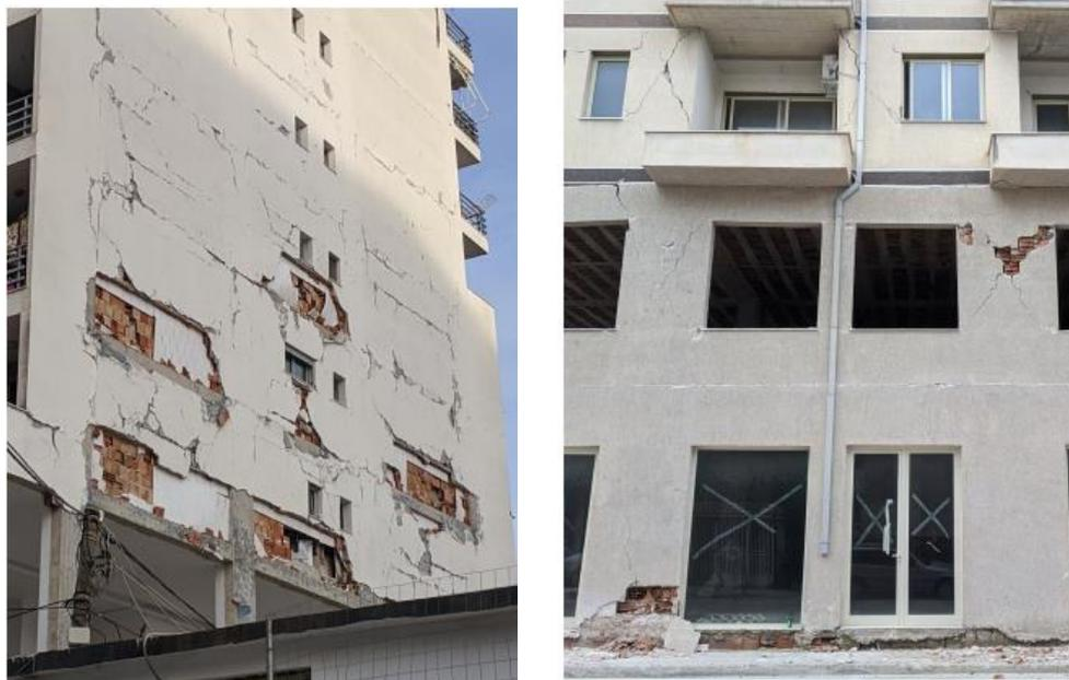
Fig. 2.7 – Damage on buildings in Durrës (McKenney, 2019)
