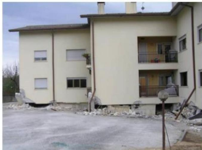
Fig. 2.34 – Three-storey RC structure in Italy that failed due to soft-storey mechanism (Verdarama, G.)
