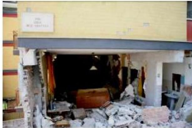
Fig. 2.3 - Example of damage owing to frames arranged only in one direction (Marazzi et al., 2011)
