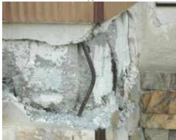
Fig. 2.4 - Insufficient reinforcement resulting in buckling of vertical rebars (Marazzi et al., 2011)
