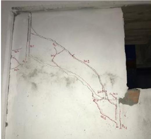
Fig. 3.19 – Cracks along the infill wall main diagonal (ISAAC technical report, 2020)
