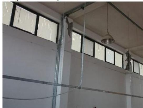
Fig. 2.9 – Damage due to short-column mechanism (Leti and Bilgin, 2021)
