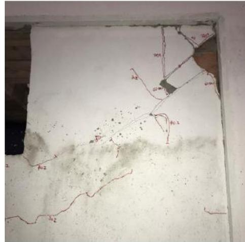
Fig. 3.20 – Crushing at the infill wall corner (ISAAC technical report, 2020)
