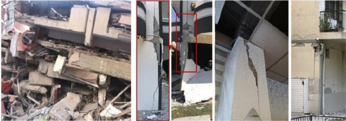
Fig. 2.14 – Strong-beam and weak-column mechanisms (Koçer and Ünal, 2022)
