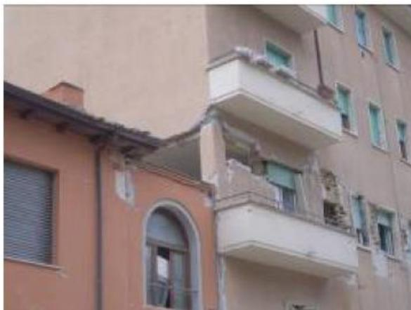
Fig. 2.2 – Damage due to design flaw of buildings without coinciding floors (Marazzi et al., 2011)
