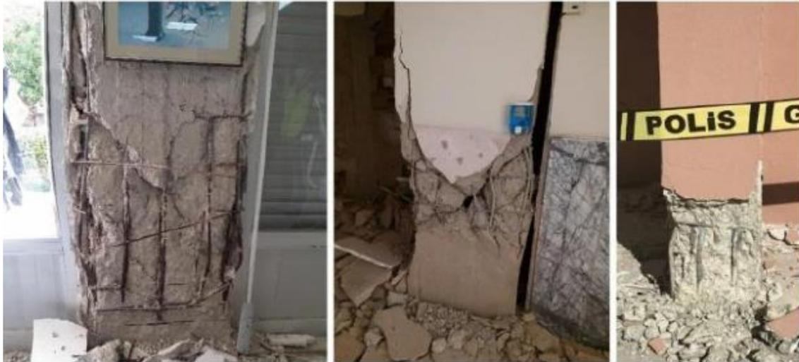
Fig. 2.13 – Column damages (Koçer and Ünal, 2022)
