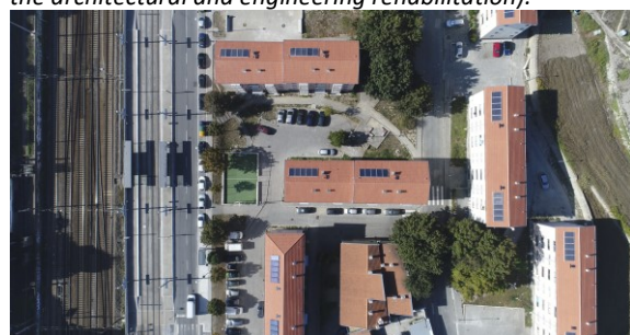
Figure 13: Solar panels view at Machado Vaz Neighbourhood (after the architectural and engineering rehabilitation).
