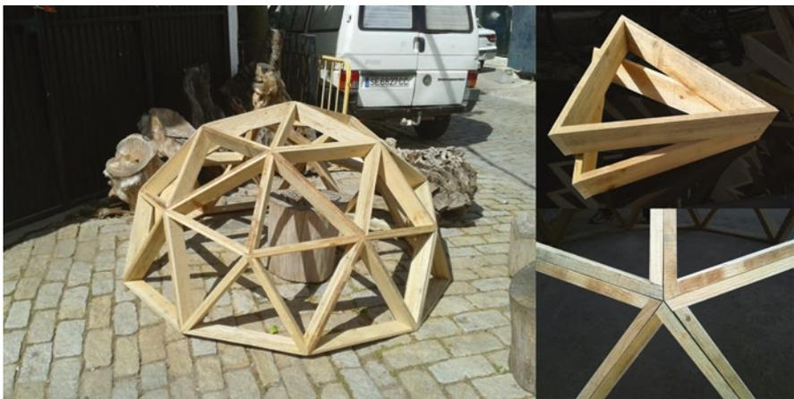
Fig. 7.4 Hemispheric structure, module, and vertex detail in the *GoodKarma* constructive system
