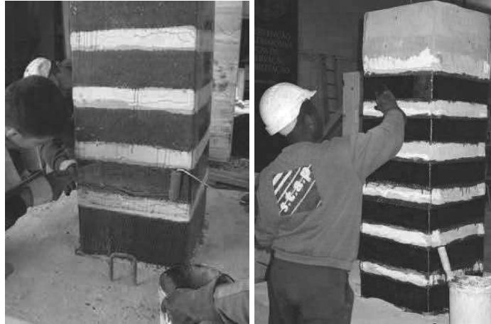
Figure 3: Pier reinforced with CFRP.
