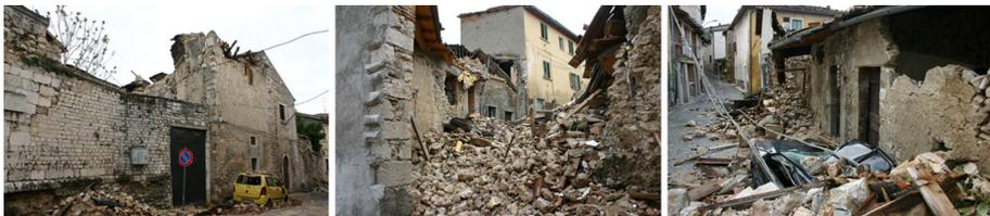
**Fig. 1** Unreinforced stone masonry buildings damaged after the 2009 L'Aquila earthquake
