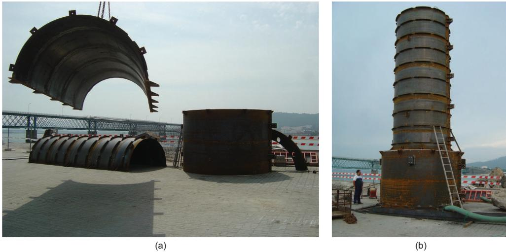
Figure 7. Formwork components and erected formwork
