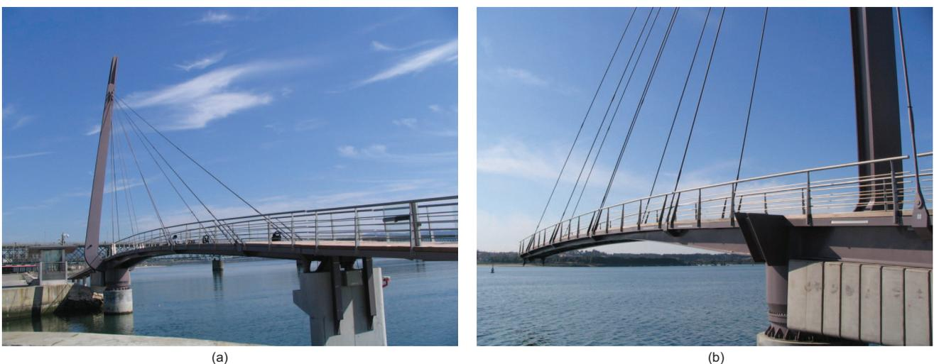
**Figure 4.** Images of the footbridge in the two operating positions: (a) closed, for use by pedestrians; and (b) open, to allow the entrance of sailing boats into the marina
