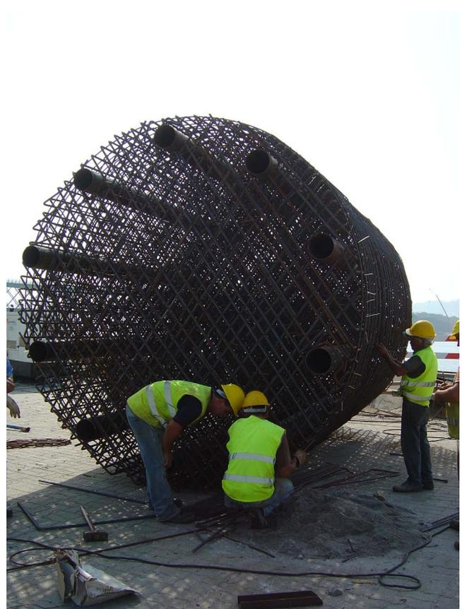
Figure 8. Lower reinforcement
