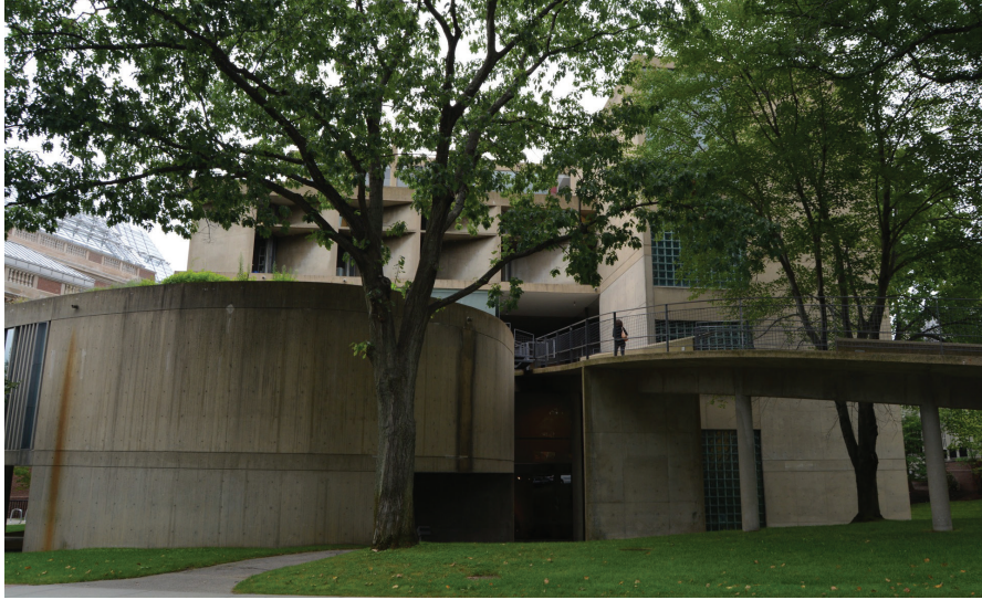
XXIII Carpenter Center for the Visual Arts, Cambridge, Boston, 1961, Le Corbusier.
