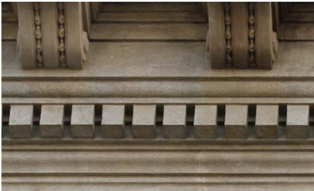
Figura 29 – Denticulos fachada lateral, 2019
