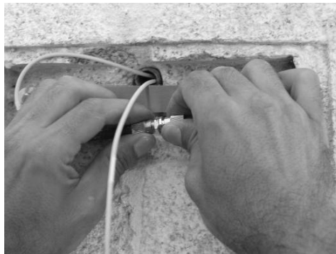
Figure 18. Coupling: (a) fusion splice; (b) butt-joint connection.
