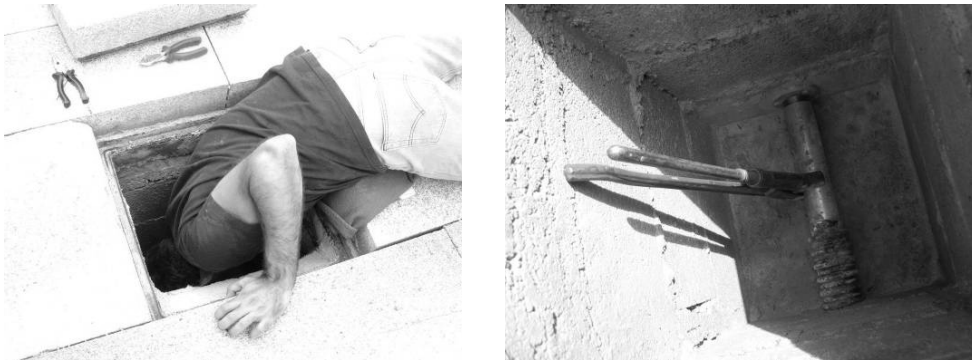
Figure 20. Installation of invar wire for Long Gauges: (a) access to the sensors; (b) used wrench.
