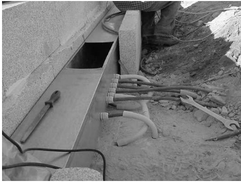
Figure 17. Distribution of fiber optic cables along the bridge: (a) metallic duct; (b) fiber optic cabling.
