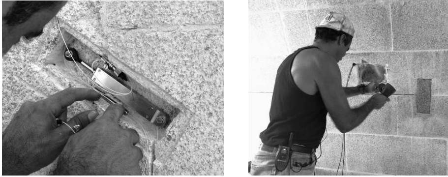
Figure 21. Installation issues: (a) LPDSs in small cavities; (b) composite strain sensors in the intrados .
