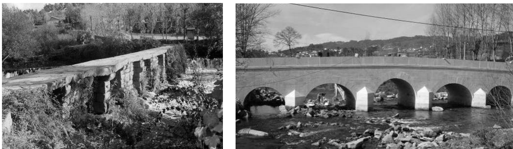
Figure 1. The Vila Fria (a) old and (b) new stone masonry bridge.
