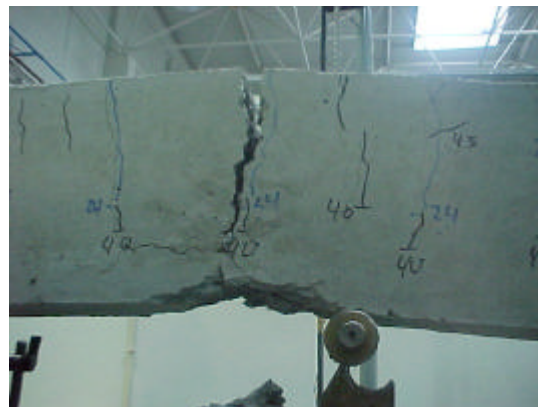
Fig. 7. Rupture of a reference beam.
