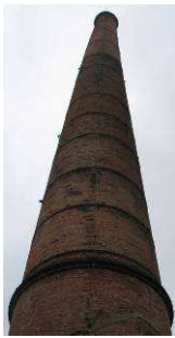
Figure 5: Chimney deformed shape
