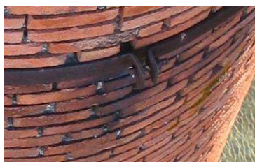
Figure 11: Corroded ring connection
