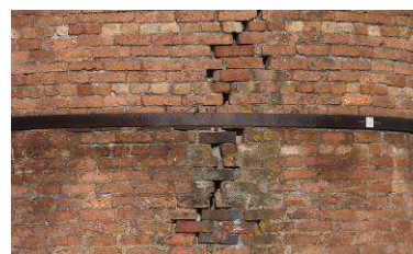
Figure 12: Crack crossing a corroded ring
