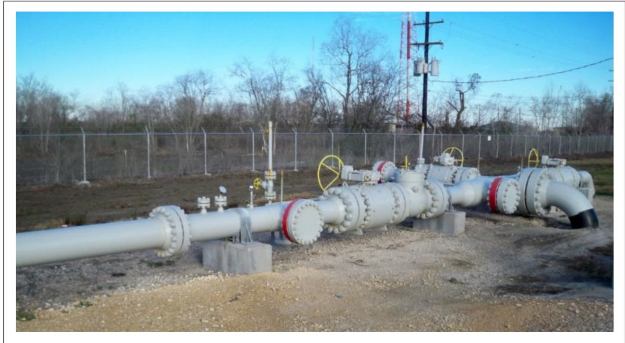
**Figure 20:** 400 mm diameter commercial CO<sub>2</sub> pipeline at above/below ground transition, [12].
