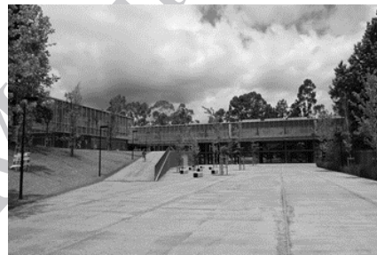
Fig. 6 Complete transformation of the school image. Escola Secundária de Lousada, Architect José Manuel Carvalho Araújo (2012) © André Santos
